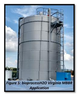
bioFAS™ Moving Bed Biofilm Reactors (MBBR) are commonly used for industrial wastewater treatment applications and provide pretreatment and removal of organics in wastewater streams. MBBR systems can effectively be integrated with industrial and municipal treatment systems for BOD removal, nitrification and denitrification. These systems are durable against toxic shock loads and are easy to operate and maintain.
